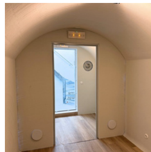
Vaulted concrete module
